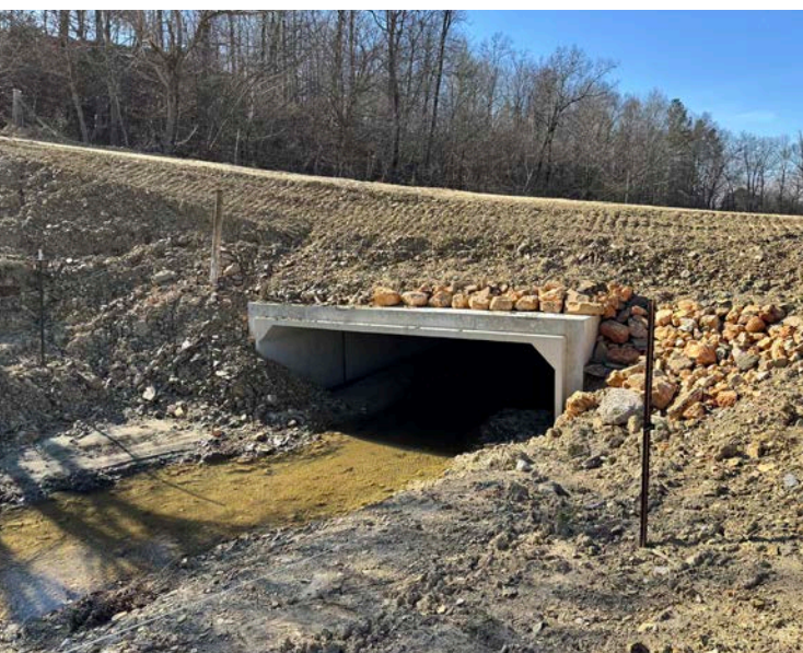
A newly completed concrete culvert, shown shortly after construction and ahead of revegetation.
