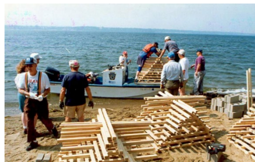
Figure 68. Porcupine Cribs for Fish Habitat
