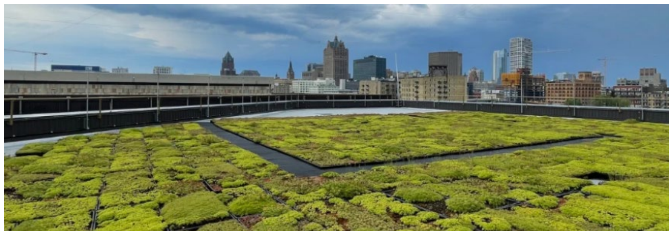
Figure 86. Green Roof in Milwaukee
