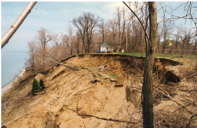
Figure 62. Failing Bluff Along Lake Erie, PA, Coastline
