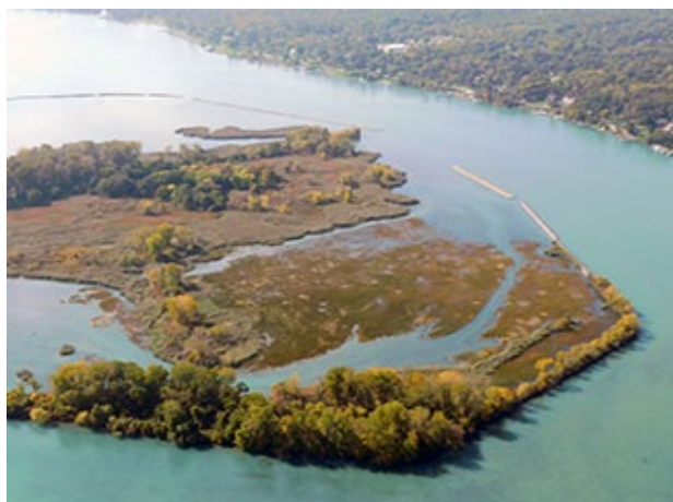
Figure 47. Pointe Mouillee Marsh Restoration
