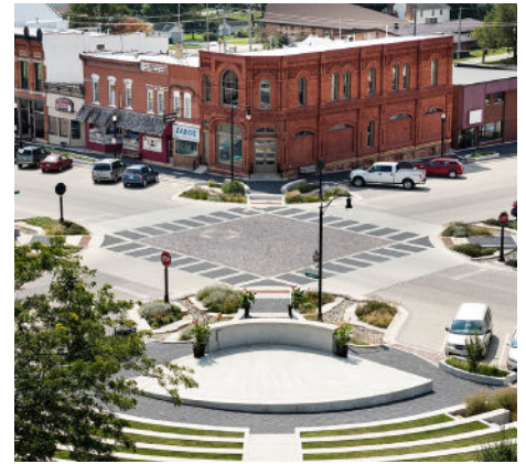
West Union, Iowa Green Streets, Amphitheater & Geothermal System
